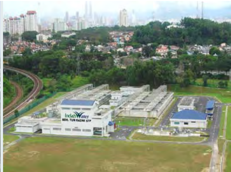
After - Bandar Tun Razak Mechanised STP
