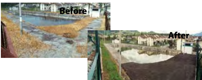
Most treatment plants handed over to Indah Water were found to be totally neglected and posed safety and environment hazards.
