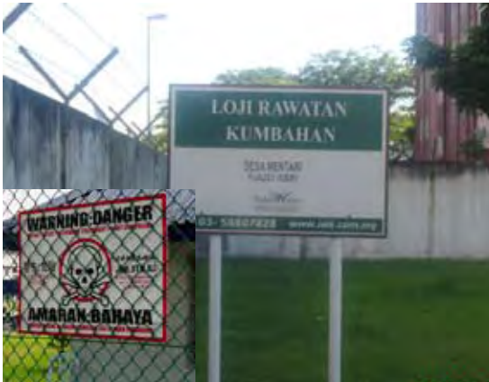
Adequate safety & warning signages erected at Indah Water Treatment Plant
