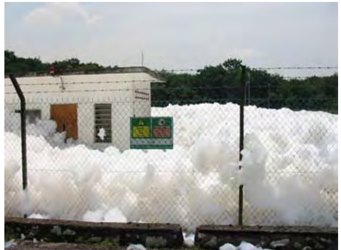
Illegal industrial detergent discharge into STP
