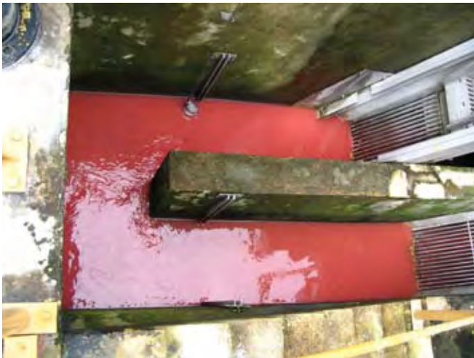
Suspected illegal discharge of die/paint
