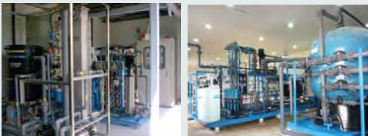
Application of Continuous Submerged MF (CMF-S) followed by Reverse Osmosis (RO) membrane for waste water reclamation
