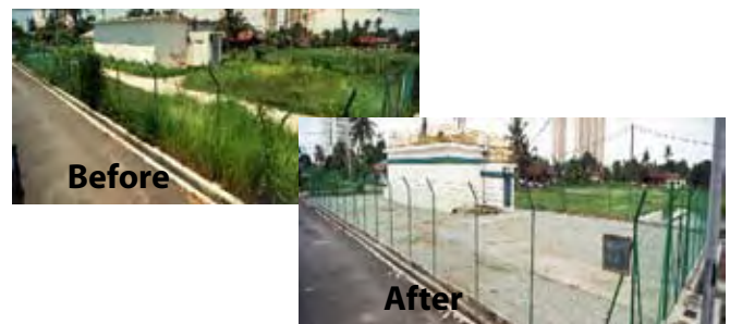
A number of plants were found to be inaccessible for maintenance due to overgrown vegetation. This contributed to the non-performance of the treatment plants.
